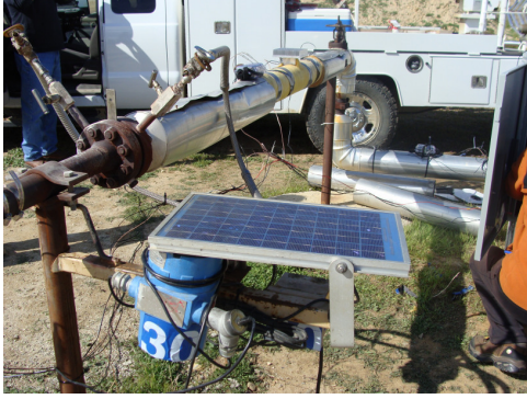
Figure 13. Invasive flow sensing with solar panel for power.
